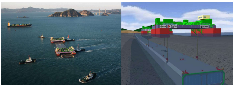
Fig. 3: Tunnel element at project location and during immersion (Busan Geoje, South Korea)
