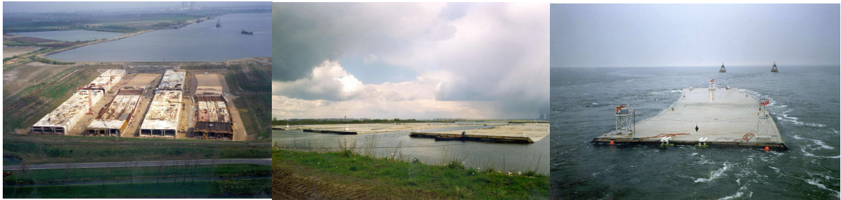
Fig. 2: Tunnel elements in casting basin, in flooded casting basin and during offshore transport (Piet Heintunnel, The Netherlands)
