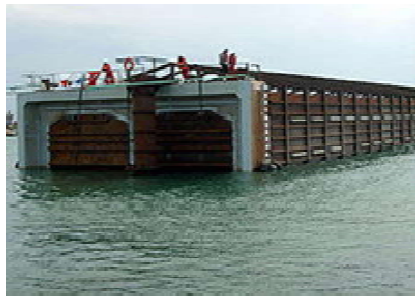
Fig. 8: Marmaray Crossing, Turkey
