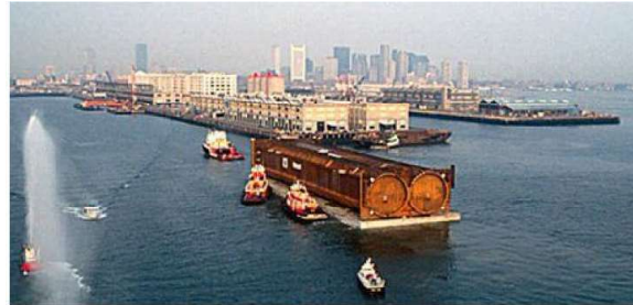
Fig. 6: Transport of steel tunnel element (Ted Williams tunnel, Boston, US)
