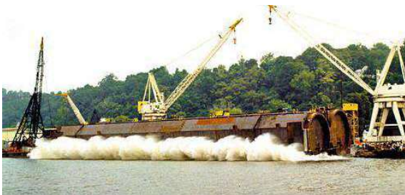
Fig. 5: Launching of steel tunnel element
