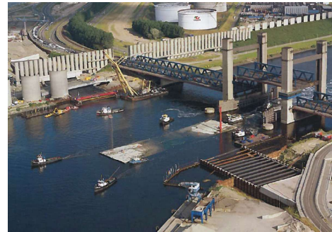
Fig.13: floating tunnel element arriving at site and passing under existing movable bridge
